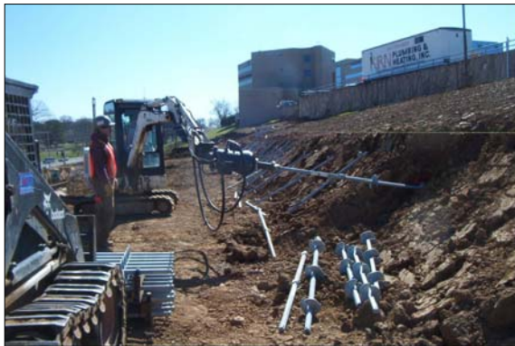
Screw installations revealing lead helical square shaft anchors ready for installation.
