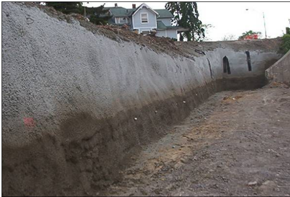
Second stage completed.
