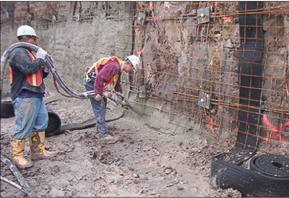
Shot Crete spray placed on readied wall.
