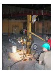
Hand held units for interior works have similar capacity. However they can be carried in sections and snapped together in restricted areas. That feature allows use in such tight spaces as, closets, small bathrooms and crawlspaces.
