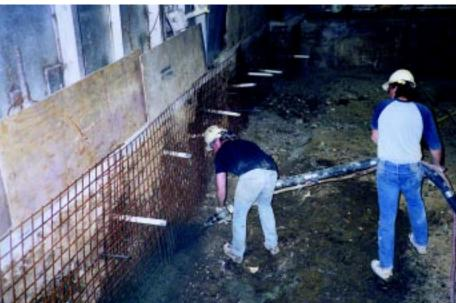
ing plates, and a shotcrete covering was applied. The anchors were installed at a torque reading of 6,000 ft.-lb. which converts to a 60 kip ultimate capacity. Applying a 2.0 safety factor yielded a 30 kip working load.
