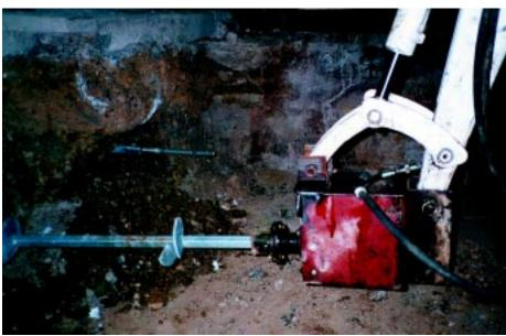
Screw anchors were installed. The excavation and installation process was performed in three equal lifts of 4 ft. each, with each row consisting of 14 anchors.
