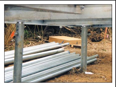
Eight Type HS 3½-inch diameter Chance Instant Foundation Screw Piles were installed. To achieve design requirements, 7 ft. lead sections with 10- and 12inch-diameter helices and 78inch-long plain extension sections were used. A special pile cap manufactured by Chance was used to connect each pile to the superstructure.
