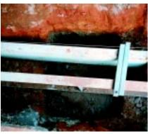
and from 50 to 55 ft. along the pile row closer to the river. All anchors were installed to 5,300 ft.-lb. of torque.
