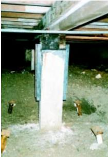
depth of the anchors was approximately 18 ft. with a minimum average installation torque of 1,500 ft.-lb. from a Chance 2500 ft.-lb. portable drive unit.
