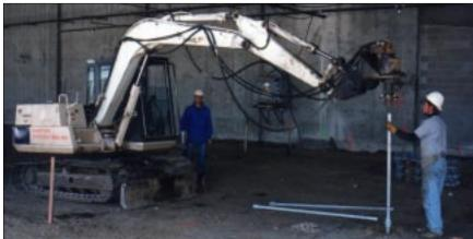
section of I-880 that collapsed during the 1989 Loma Prieta earthquake. The original floor was a floating slab which could subject the restaurant's contents to considerable damage during an earthquake. A slab on grade beams supported by Chance anchors was chosen to mitigate potential seismic damage. Because the anchors were cast in grade beams, lateral restraint was supplied by the parking garage's foundation.
