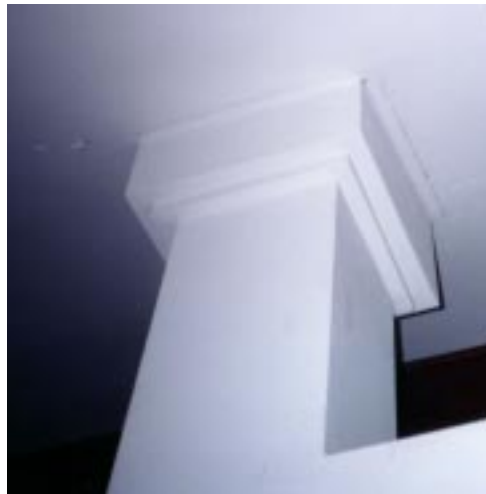
Gap is closed after lifting slab.
