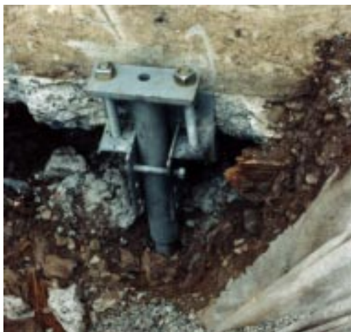
HELICAL PIER underpinning bracket
