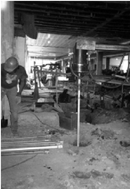
Chance anchor being installed in slab area on a 10' grid
