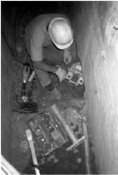
Underpinning bracket being assembled onto Chance HELICAL PIER® Foundation Systems anchor and under utility vault
