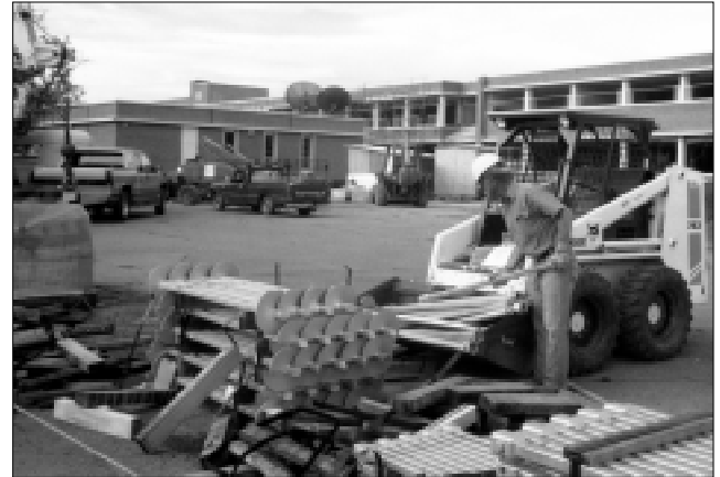
Screw anchors and extensions being moved into the Montrose High School
