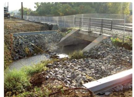
Stone riprap was placed at both abutments and along the channel. A gabion wall [wire mesh encased riprap] was installed along the fence line to act as a retaining wall.
