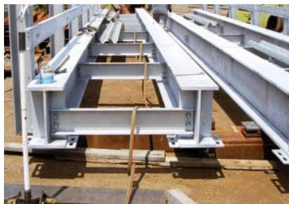
The bridge superstructure was constructed of steel stringers with diaphragms equally spaced along the length of the bridge. The bridge was prefabricated in two 8 foot wide sections, each measuring 39 feet long.
