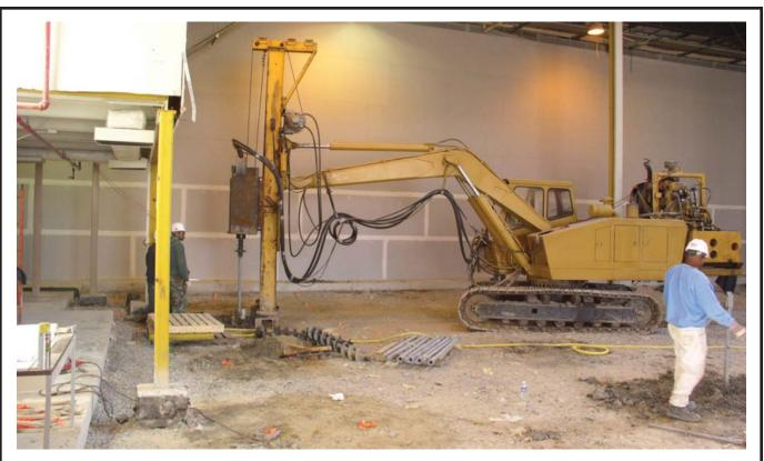
of the HPM, soil is displaced to create a void around the square shaft. Flowable grout immediately fills this void from a reservoir at the surface.
