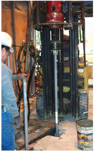
lead section consisted of three helical plates: 10-, 12- and 14-inch diameters. Extension sections were added until the helices reached competent loadbearing soil. All square-shaft helical pier components were hot-dip galvanized.
