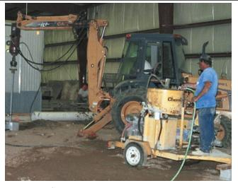
structural floor design and required pile layout and capacities. Calculus selected the HELICAL PULL DOWN® Micropile because it was the most cost-effective solution providing the required 100-kip-per-pile ultimate capacity.
